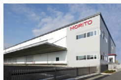
MORITO KANTO LOGISTICS CENTER
